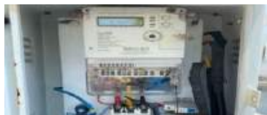
Gambar 3. Kwh Meter IBAP Banjar Kemuning
